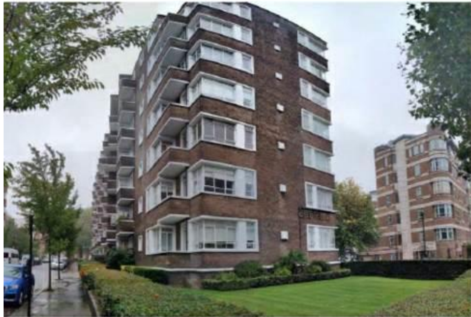
View of southern elevation from Prince Albert Road
