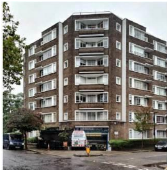
View of northern elevation at the junction with Newcourt Street and Culworth Street
