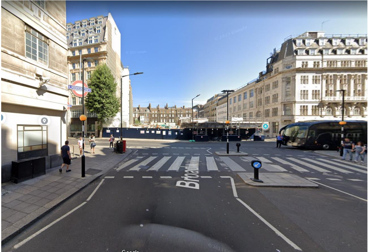
40 Broadway post demolition
