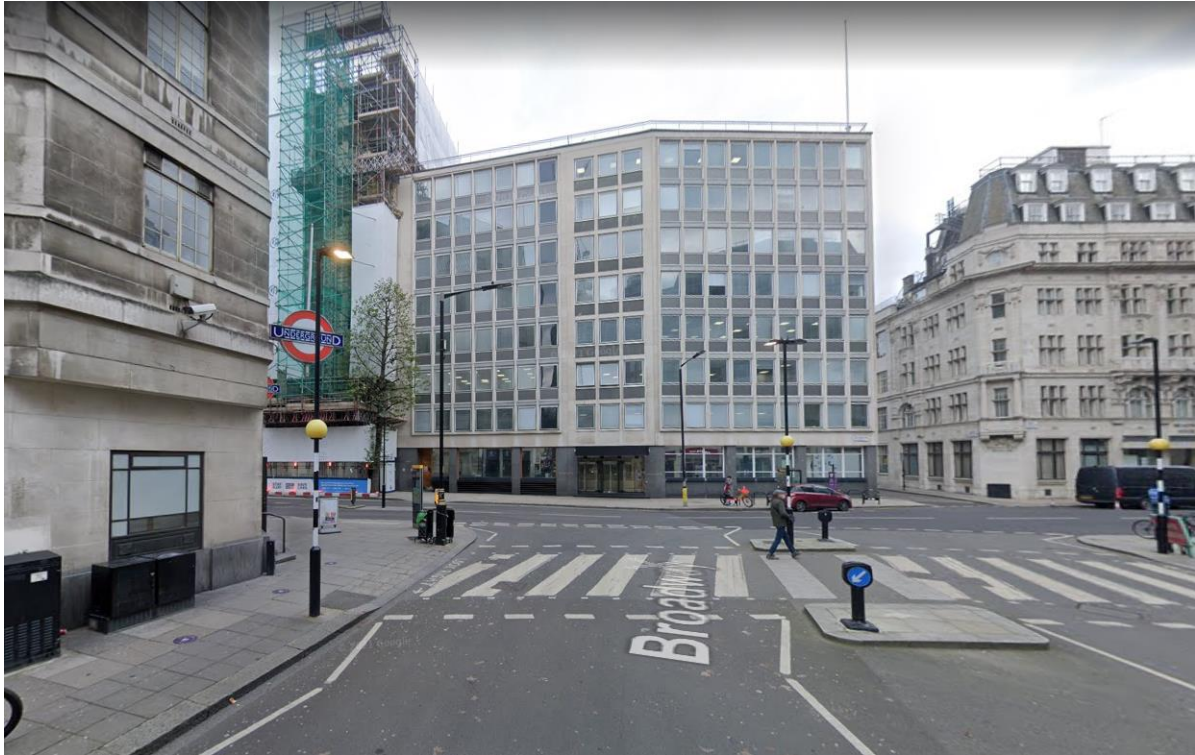
40 Broadway elevation pre-demolition
