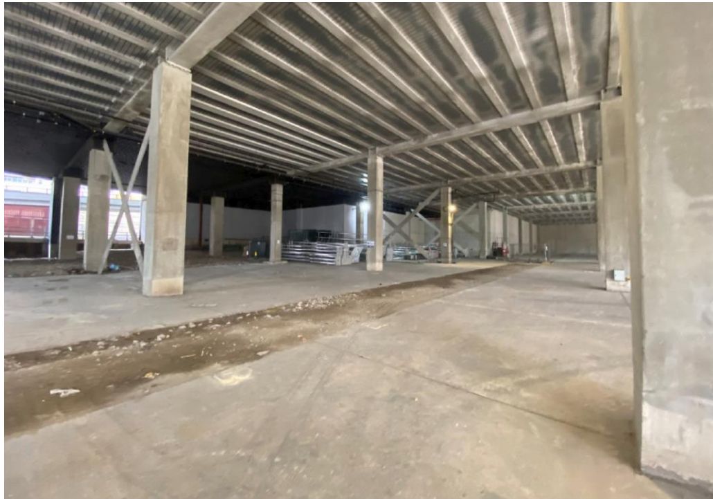
View east within "Crossrail box"
