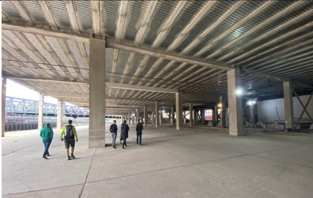
View west within "Crossrail box"
